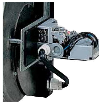
Air damper adjustment
